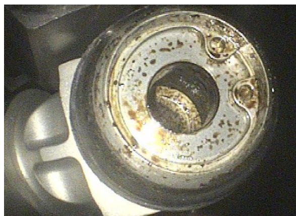
Figure 11 – Black Deposit in Fuel Gas Nozzle
