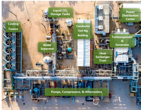
50 MW th Demonstration Facility and turboexpander [NET Power, 2024]
