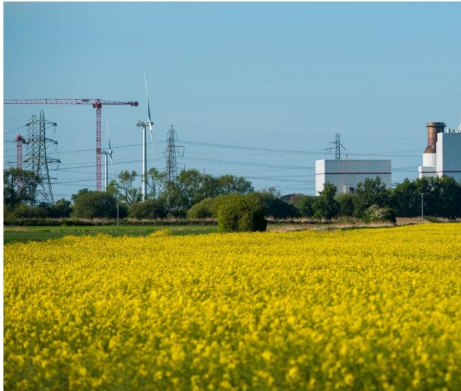
The Keadby 1 power station. (Photo: Stuart Nicol / SSE Thermal)
