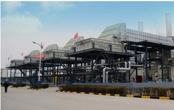
Figure 15 – Titan 130 conventional combustion gas turbine packages operating with up to 65% hydrogen [33].
