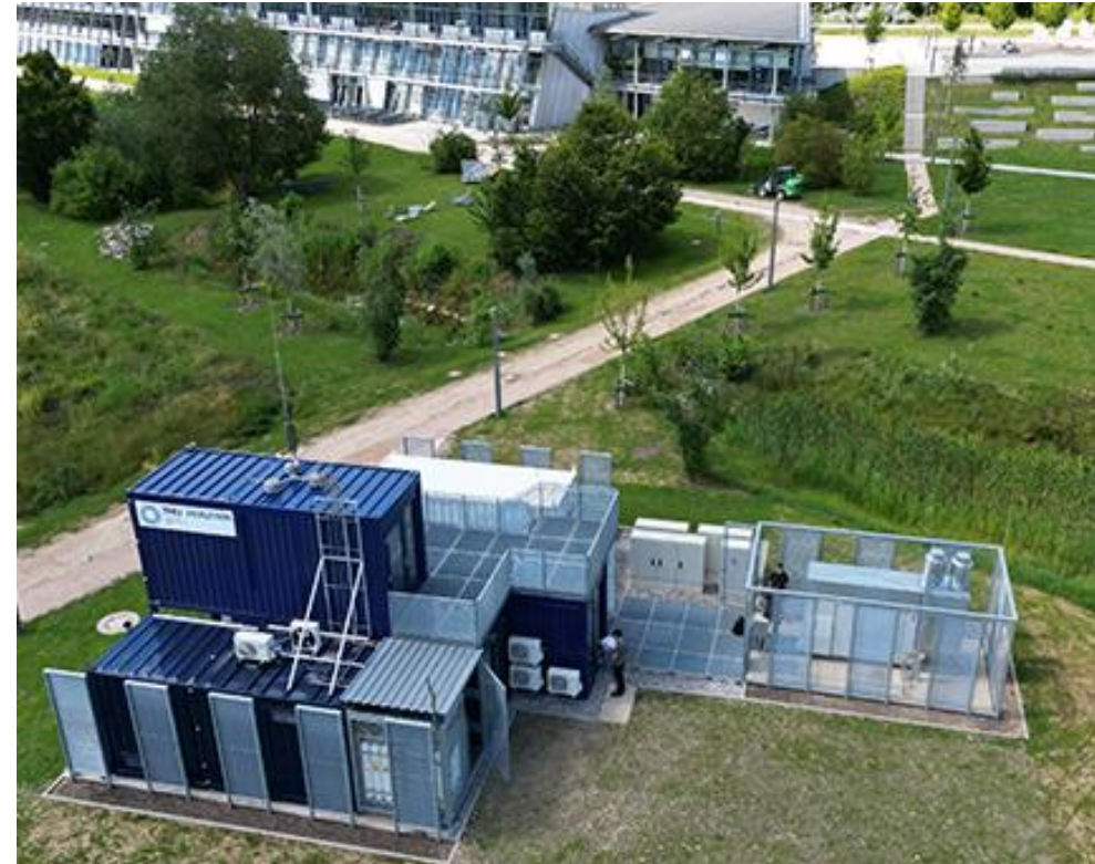
Energy storage and conversion system with battery storage, electrolyser, hydrogen storage and gas turbine in the Energy Park of TH Ulm
