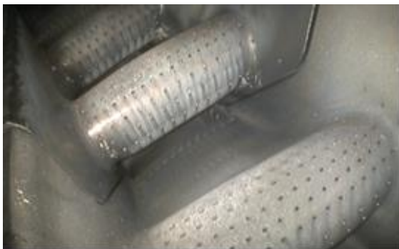
Figure 10 A S1N Borecope inspection
