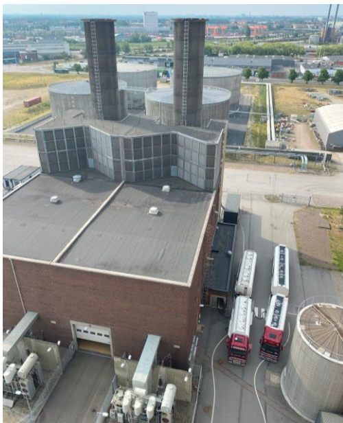
Fig. 2 Two 50 m 3 tankers supplying HVO during the ÖVT V93.0 GT field trial
