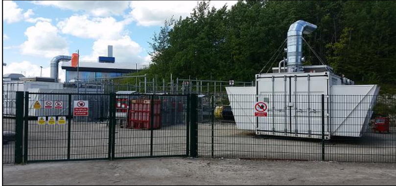
Internal combustion engine running on H 2 /NH 3
