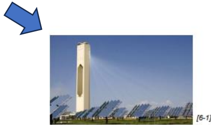
Concentrated Solar Power
