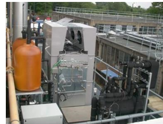
Gas cooler test facility
