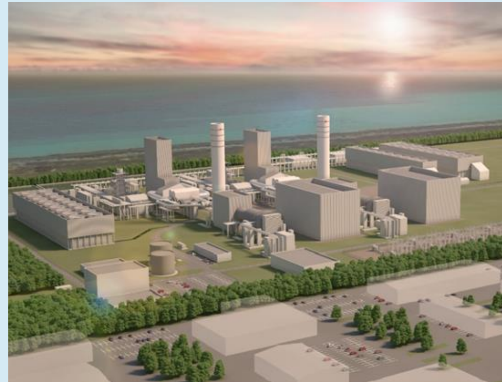
Typical impression of two 1X1 H-Class CCGT with post-combustion carbon capture, Adapted from [5]
