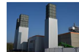
Combustion Test Center in Berlin
