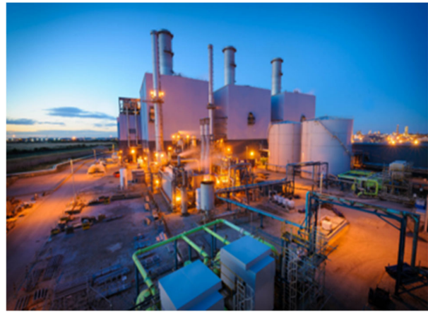
Fig. 19 Saltend power plant in the UK (Humber)
