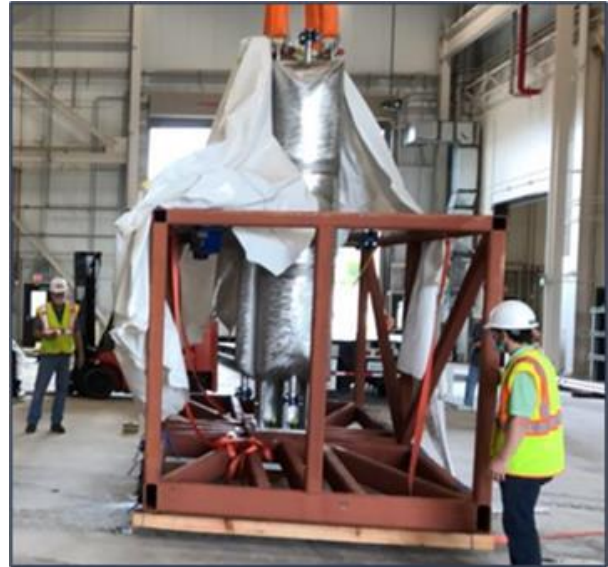
Figure 10 Compact LTR s\text{CO}_2 recuperator delivered to facility
