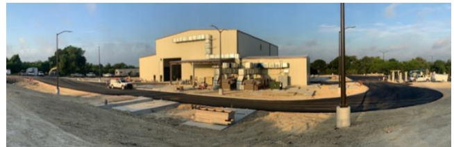
Figure 3 – Side view of SwRI GPTF building March 2020
