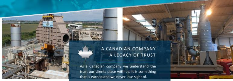
INNOVA Global was selected by Siemens to design, fabricate and install a CO \ NOx reduction system into an existing RB211 system. The project required that Innova model the existing gas turbine & waste heat boiler system to determine the optimal location to locate the new distribution grids, CO catalyst, ammonia injection and NOx catalyst components.
