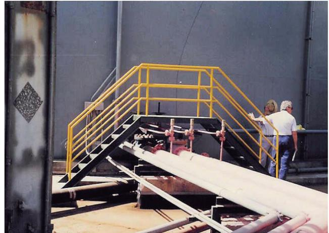
Figure 45. Poor Design of Piping from No. 2 Diesel Fuel Tank.
