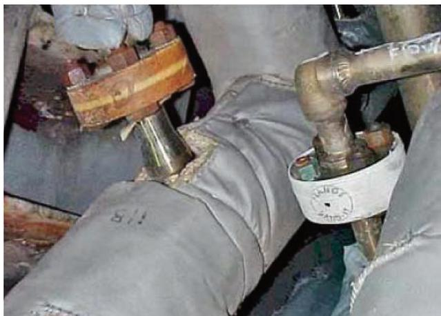
Figure 23. Flange Leak Testing. (Courtesy Flange Band-It LLC)
