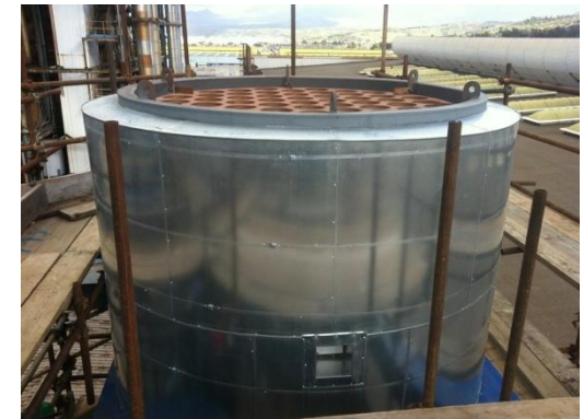
Detail of RH steam vent
