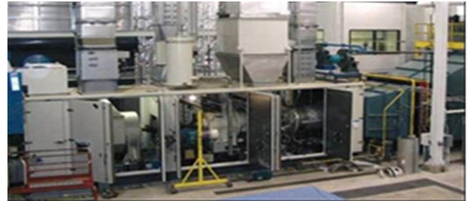
7.7MW tri-fuel gas turbine installed in a cogeneration plant in the USA
