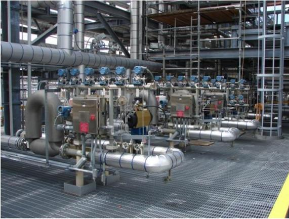
**Figure 8 - Fuel blending system hardware**
