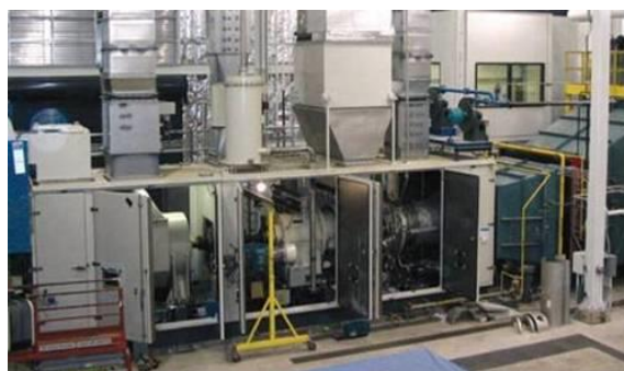
Figure 5: SGT-300 at University of New Hampshire, operating on a processed Landfill Gas
