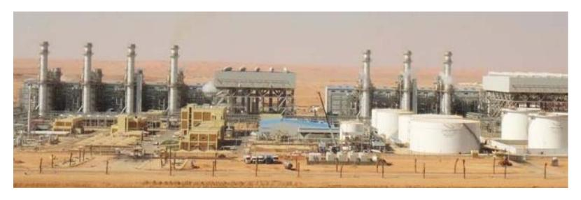
• 120 hour field test successfully performed on a 7F.04 gas turbine in Saudi Arabia; First Fclass DLN combustion system to operate on crude oil
