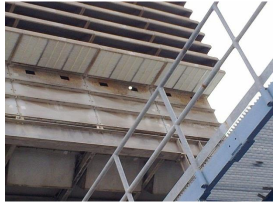
Figure 13. EPA-2 Pre-filter panels
