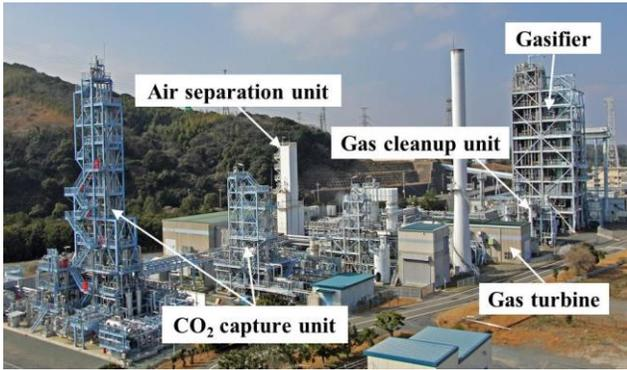
Fig. 7 EAGLE pilot plant (photo courtesy of J-POWER)
