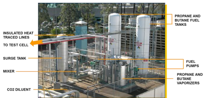
Figure 5. Fuel Blending Facility Used for Rig and Engine Testing.
