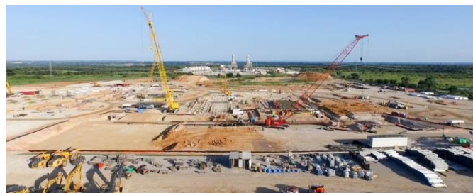
Figure 17. Exelon Wolf Hollow 7HA.02 2x1 MS Power Station under construction
