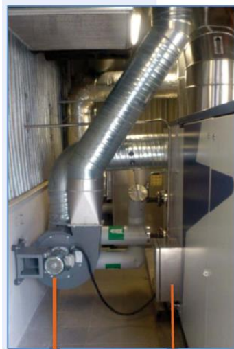
Air Evacuation Fan Biogas Safety Valves Box
