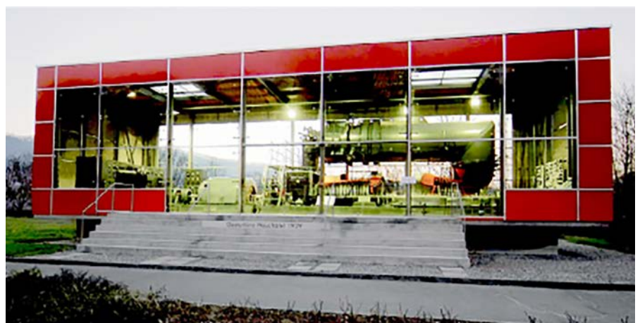
Figure 2 Neuchâtel gas turbine 1939/40, relocated to Birr, Switzerland 2007
