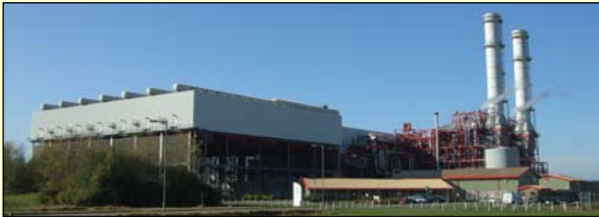
The 800 MW Sutton Bridge power station is located approximately two miles from the village of Sutton Bridge in Lincolnshire.
