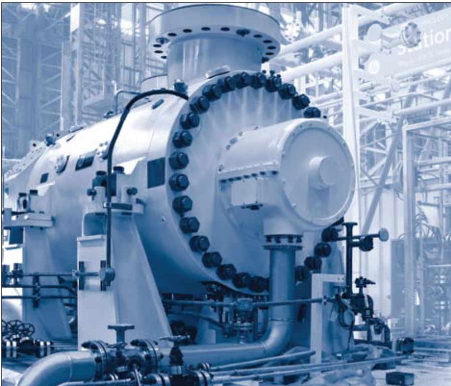
Centrifugal and axial compressors can incorporate comprehensive and integrated software packages to improve upon anti-surge control and protection.
