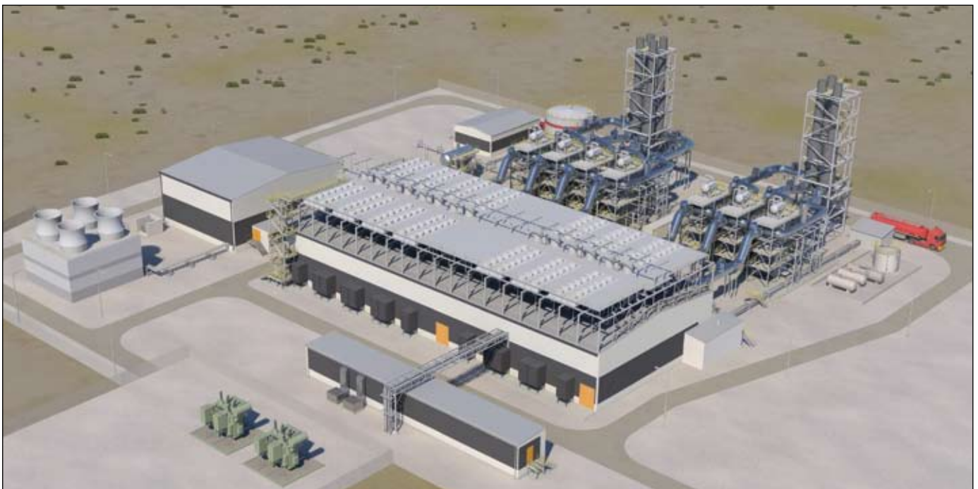
3D CAD drawing of Huinalá. The project will have an installed capacity of 139 MW generated by a Wärtsilä Flexicycle combined cycle power plant comprising seven gas engines and a single steam turbine.
