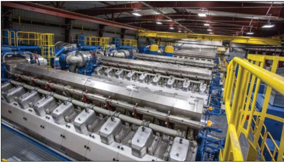
Port Westward engine hall. In a similar arrangement, all seven engines at Huinalá will be in a single engine hall.
