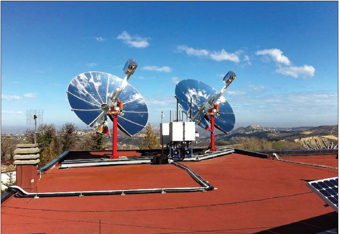
Dish/engine system. Each unit uses a parabolic dish of mirrors to direct and concentrate sunlight onto a central engine that produces electricity.
