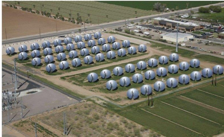
Figure 2: Maricopa power plant.
