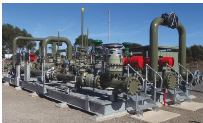
Figure 3-4: SCADA Metering station for Oil & Gas operations
