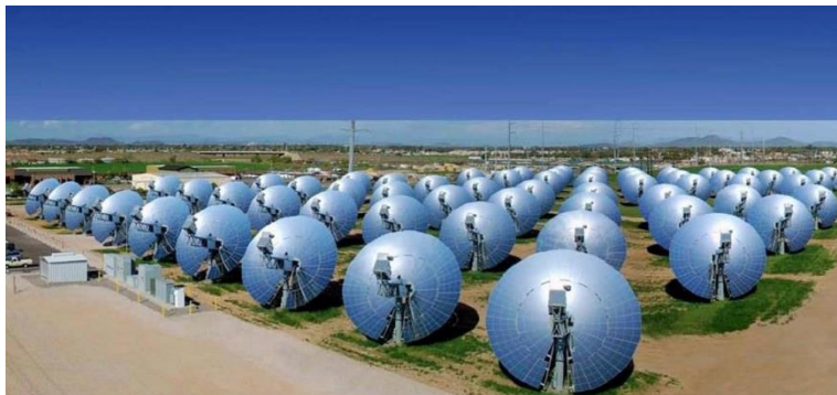
Figure 2-3: CSP dishes in farm arrangement
