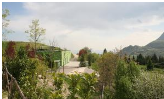
Figure 3-5: Turbec T100 units at Leafy Resort Wellness Spa for CCHP
