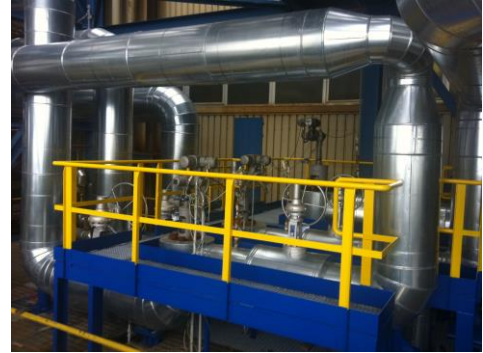
Figure 11: New warm-up HRH steam heating lines
