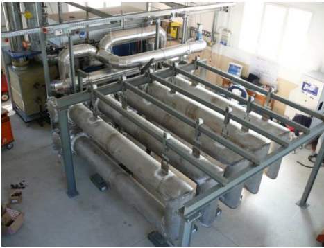
Figure 2 – The microturbine Test rig being modified for solar hybridization and storage
